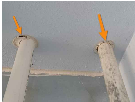
Cracked caulking
