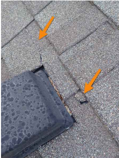
Cracked shingles
