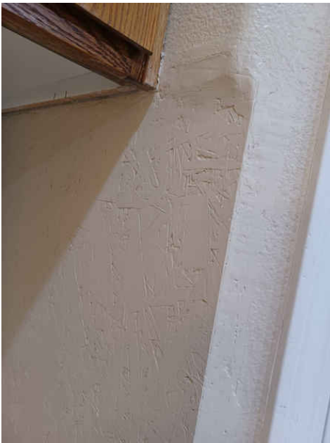
Drywall removed and OSB installed
