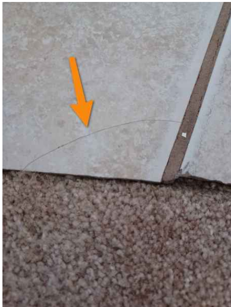
Entry to master bathroom crack in the tile
