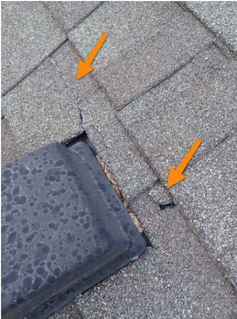
Cracked shingles
