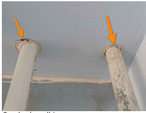
Cracked caulking
