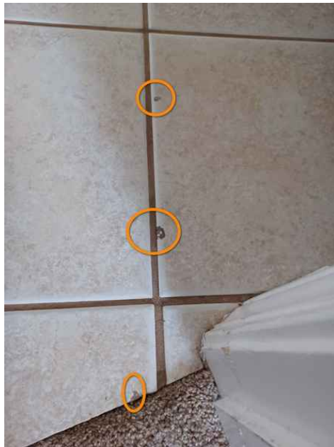
chips in the tile in the master bathroom
