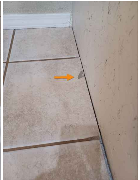
Chip in the tile in the refrigerator area
