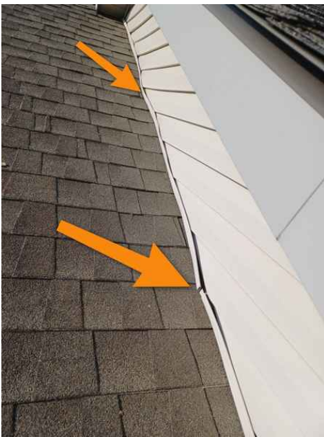
Warped siding and separated trim piece
